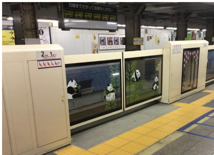
Platform Doors on Ginza Line (Source Tokyo Metro)
